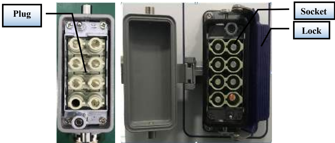
b) The picture of 6kW / 8kW / 10kW / 12kW power port plug / socket.
